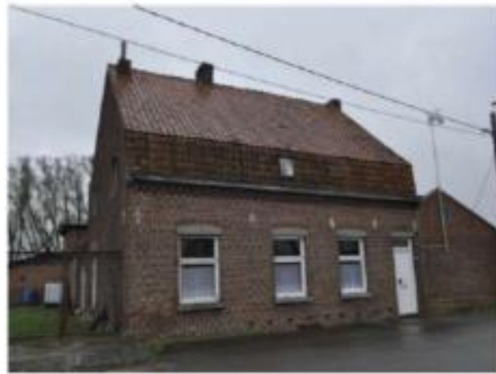
(a) Front facade, before renovation.
