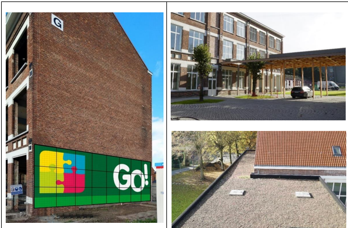
Figure 4. Left: Illustration of the green wall on the school building. Top right: side view of the awning from the playground. Bottom right: top view of the awning with a green roof.
