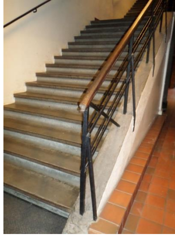
Trap in beton
